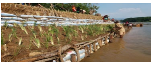
Photos: Sandbags protecting embankments; vetiver grasses strengthening embankments
