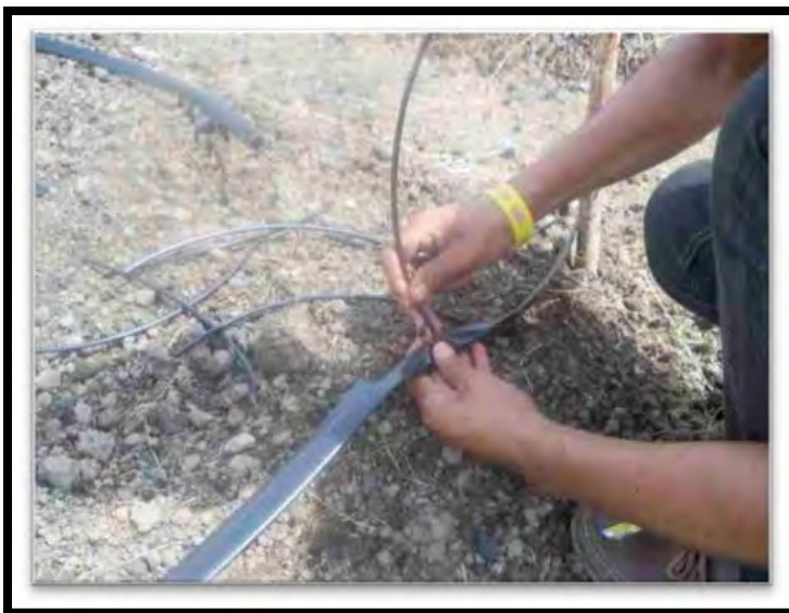
Photo 19: Connecting the Lead Hose to the Drip Tape lines
