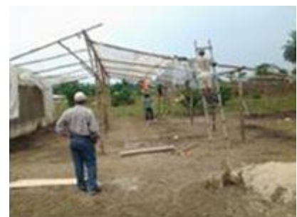
Installing the wire and PE sheet
