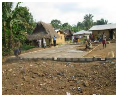
Drying floor under construction in Kuotarr Town
