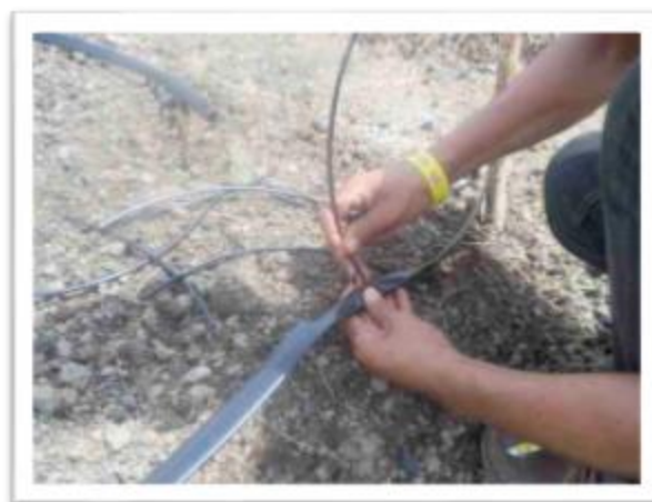
Photo 17: Connecting the Lead Hose to the Drip Tape lines
