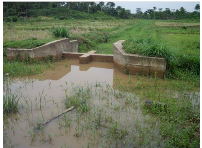
Photo VIII: Poor maintenance of the header dams
