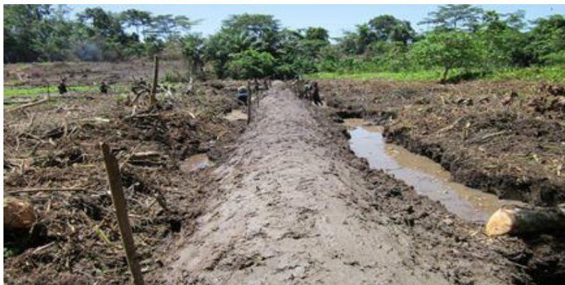
Photo XVII: A view of one of the constructed lateral bunds
