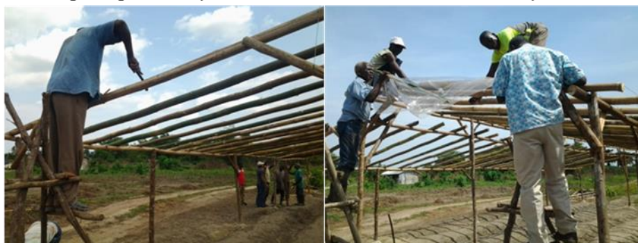
Figure 6 FED guiding Mensah production cluster farmers to install RS plastic sheet roofing
