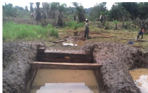
Figure 2: Completed spillway in Duaita, Jorquelleh District, Bong County.
