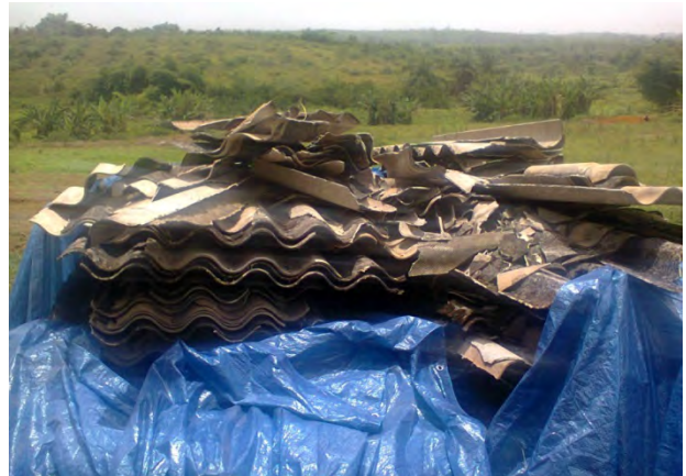
Figure 27: Asbestos being removed at BWI for the newly renovated science labs.
