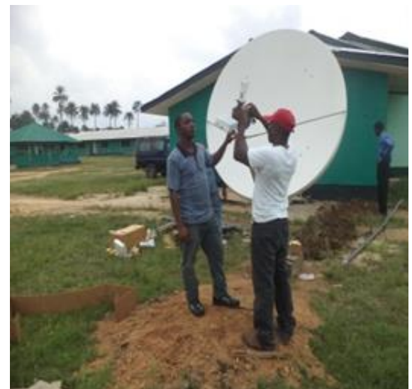
Figure 13: VSAT installation inspection at LCCC.
