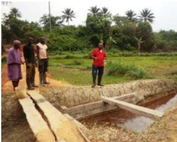
Figure 2: Completed spillway irrigation structure in Kaheniala, Lofa County.
