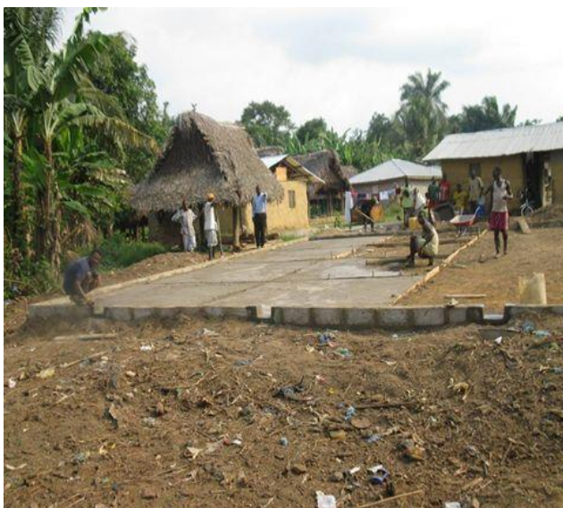
Photo 5: Drying floor under construction in Kuotarr Town
