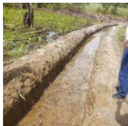
Figure 75: Payecea town lowland rice ditch being constructed.
