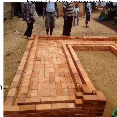
Figure 16: Zero-energy cooler being constructed in Kakata, Margibi County.
